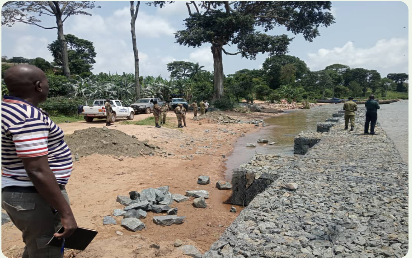
Seven people were arrested during this EPF operation for illegally erecting gabions in Lake Victoria
