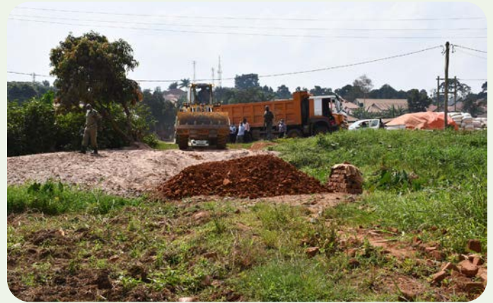
Under the supervision of EPF, Roko Construction Company removed the debris that was dumped in this wetland by one of their truck drivers
