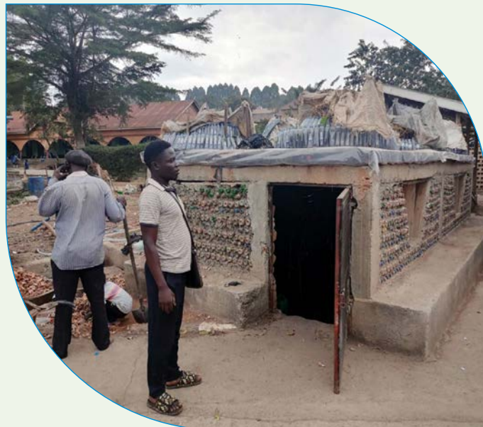
Reusing plastic in the construction of the mushroom growing facility at St. Kizito SS, Namugongo
