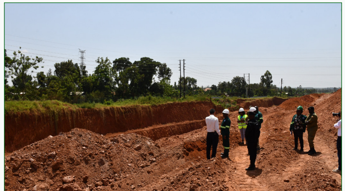
NEMA ED and staff inspecting the drainage channel being built at Sino Industrial Park
