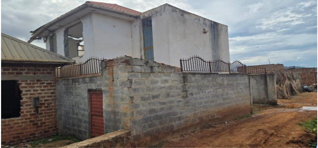
Above: Illegal structures in Kaliddubi Wetland before restoration exercise.
