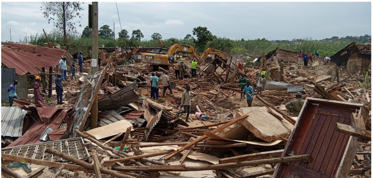
Picture showing Kawaala section of Lubigi Wetland after restoration
