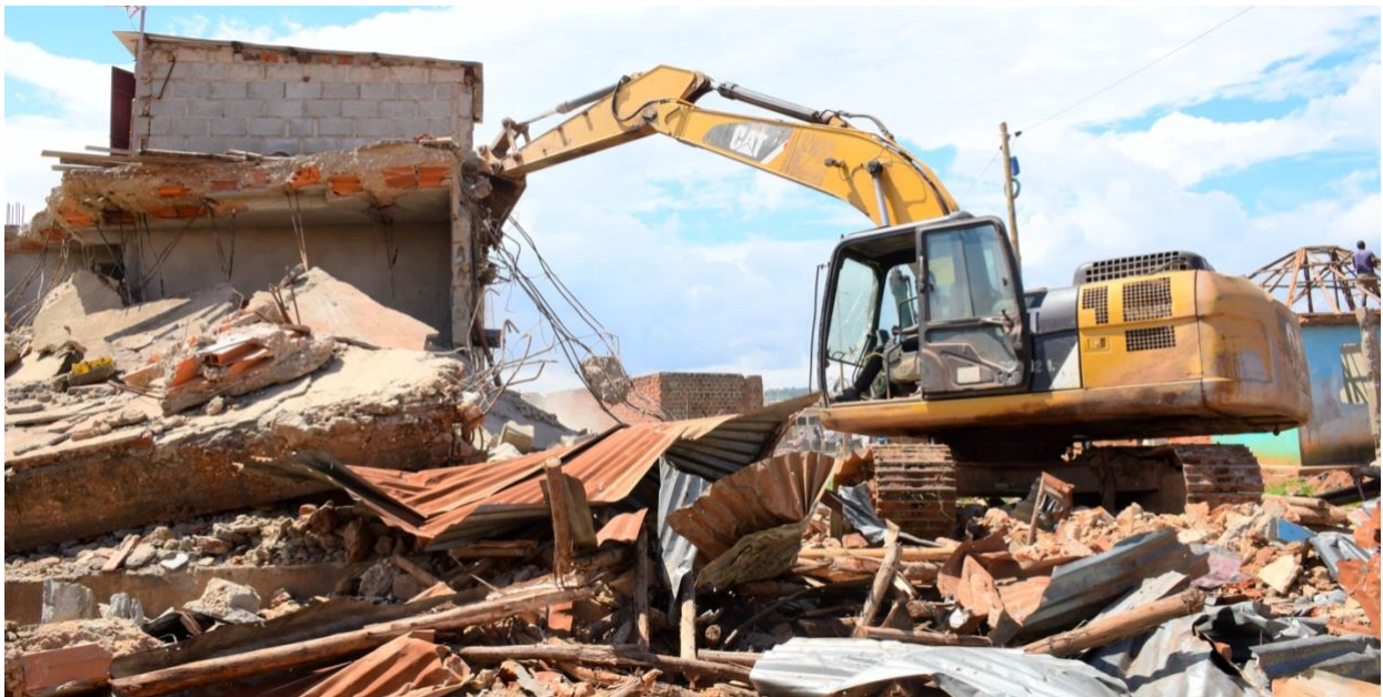
Below: Illegal structures in Kaliddubi Wetland after restoration exercise. Photo: Jeffrey Opiyo
